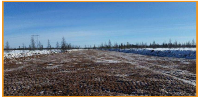
Clearing of the right-of-way and driving ice roads.
